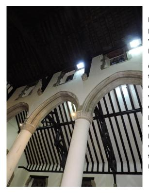
The church is current lit with metal halide flood lights located high up on the wall plate. These are effective at providing a general level of area lighting across the whole church but do not enhance or highlight any particular the features of the church.
